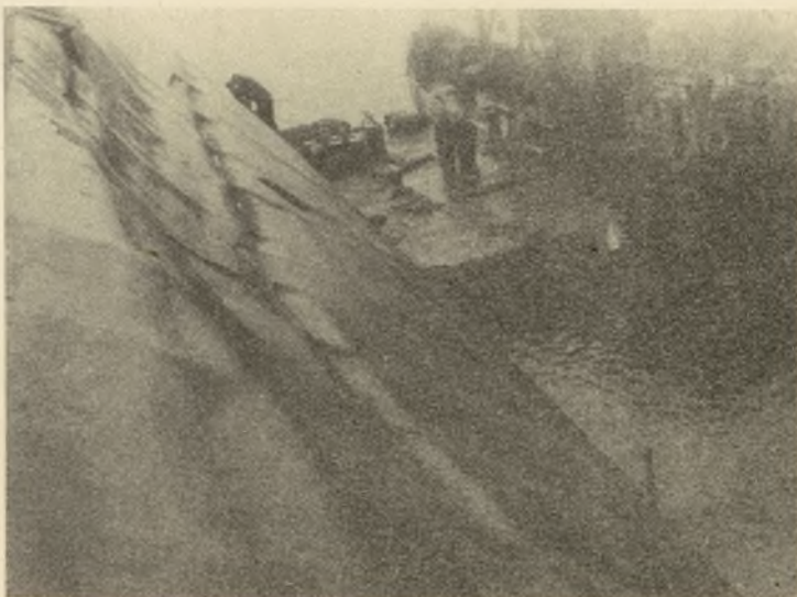
VIEW OF DAMAGE FROM 12,000 lb. NEAR MISS DENT 50 ft. LONG AND 4 ft. DEEP
