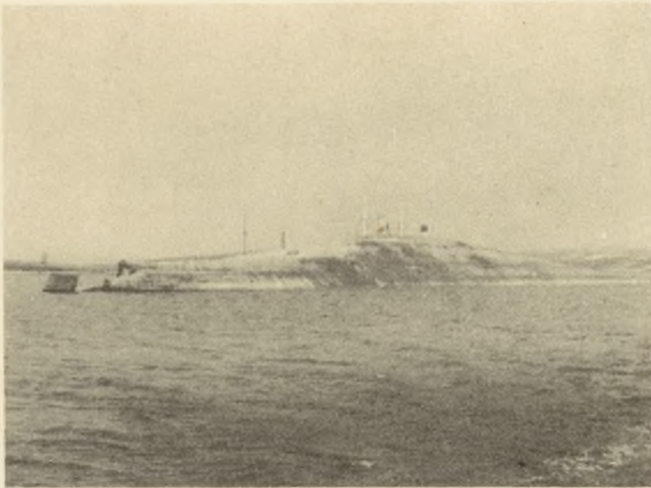
GENERAL VIEW FROM WATER SHOWING DAMAGED RUDDER
