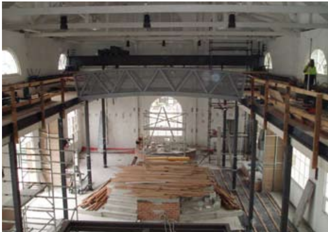
Special Exhibition Gallery under construction in the Gun Mounting Workshop building
