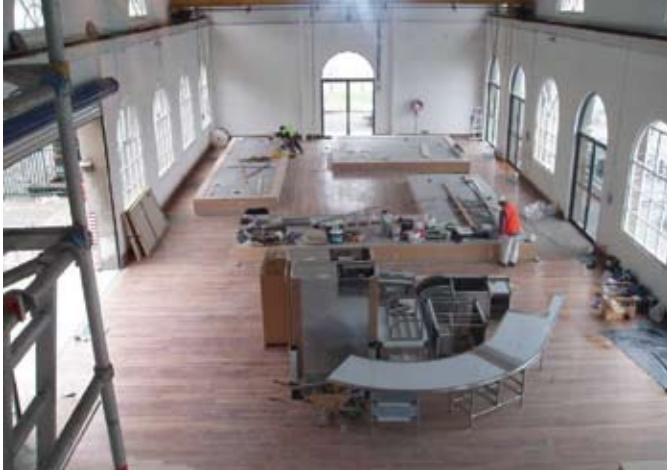
Display plinths under construction in the Gun Mounting Workshop building
