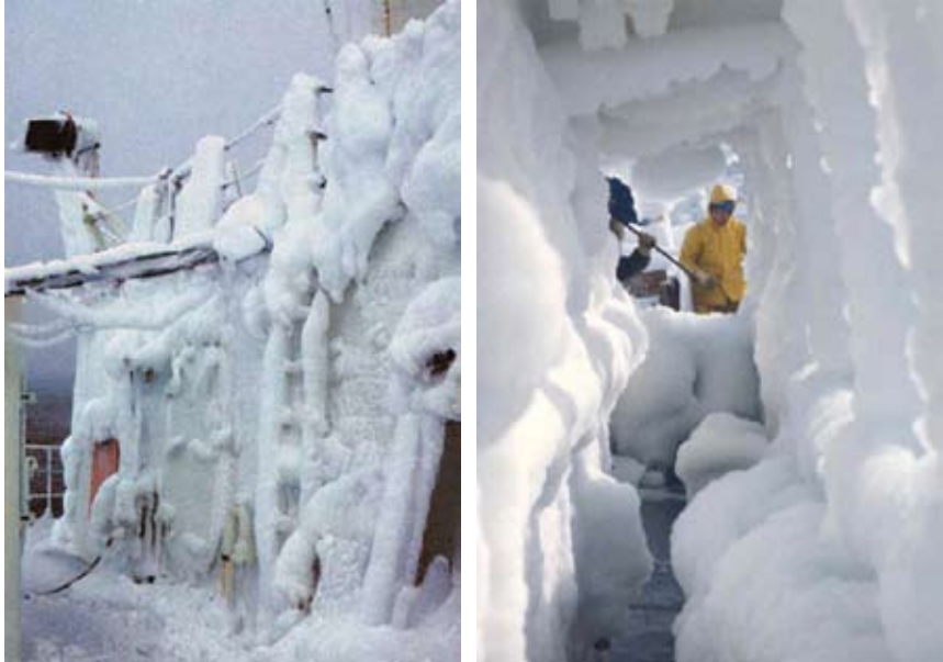
Severe ice accretion on the upper decks of a ship
