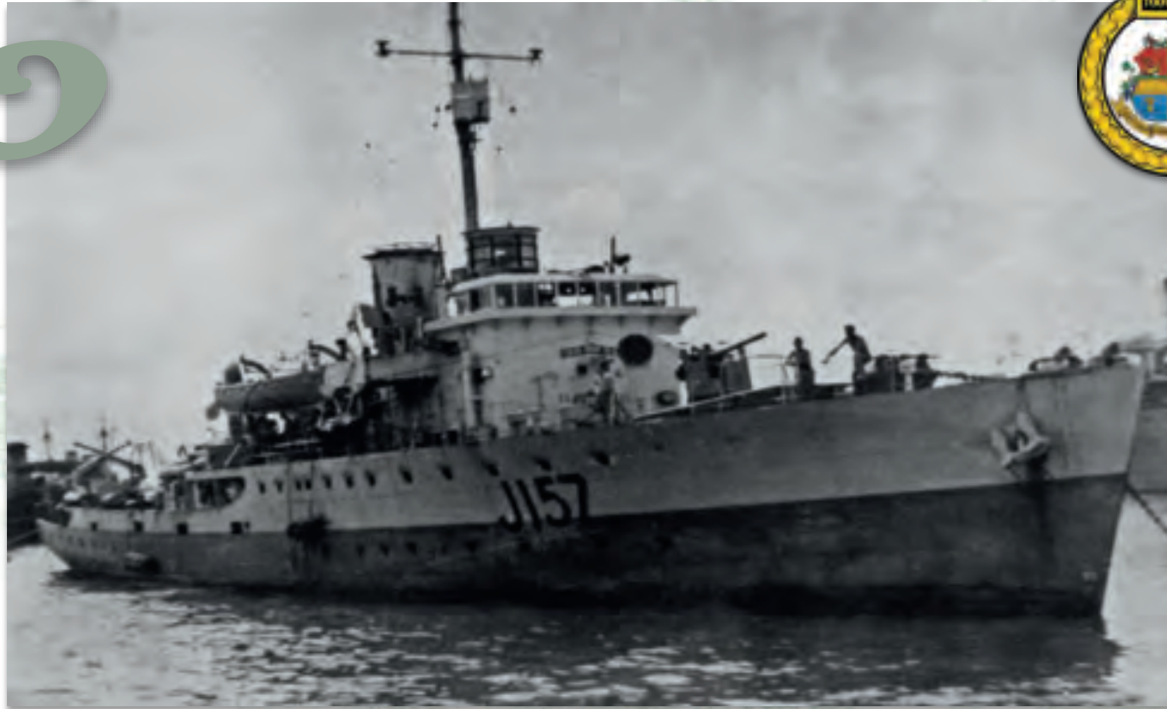
HMAS Toowoomba was built at the Walker's Yard, Maryborough, Queensland. She was named for the city of Toowoomba in the Darling Downs region of Queensland. Here she can be seen with a very early version of the 'lantern' radar housing fitted above her bridge.
