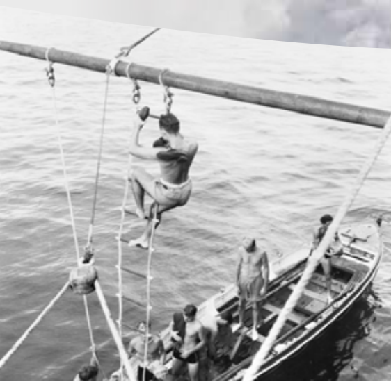
A corvette's 27-foot Montagu whaler waiting at the boat boom. (source unidentified or unestablished)
