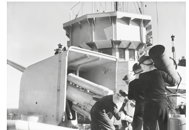
The BL 4-inch Mk IX on HMAS Maryborough . Note the higher bridge. The seaman closest to the camera is carrying the propellant charges in a special container. [AWM 009556]
