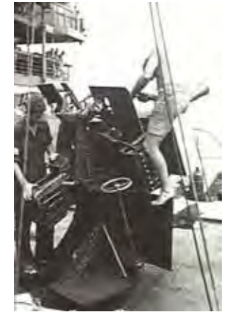
2-pdr QF Mk VIII being serviced on HMAS Bendigo . [AWM 026615]
