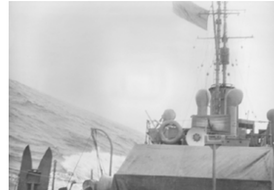
HMAS Broome showing how the Bathurst corvettes could roll. Lewis gun shield in left foreground. Note the sea is not particularly rough and the helm may be hard over turning to Starboard. The ensign is indistinct and this photograph may have been taken during builder's trials as no armament appears to be fitted. [ navy.gov.au ]
