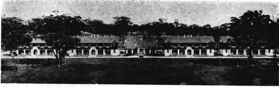
Quarter Deck and General View of Buildings.
