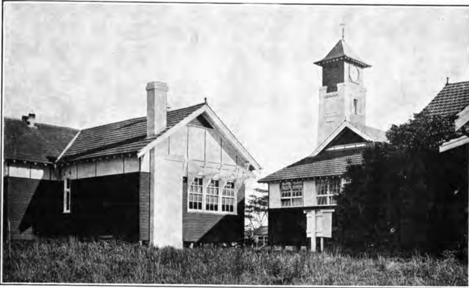
The Gymnasium from the East.
