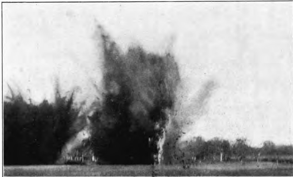
A Demolition Party at work. —Photo. by Commander Ringrose.
