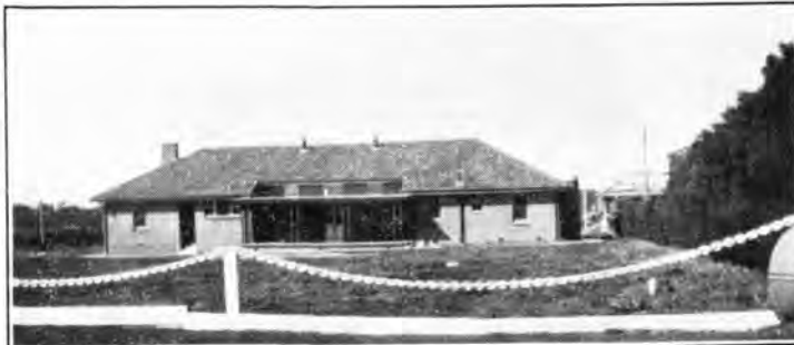
NEW HOSPITAL BLOCK—West Side.
