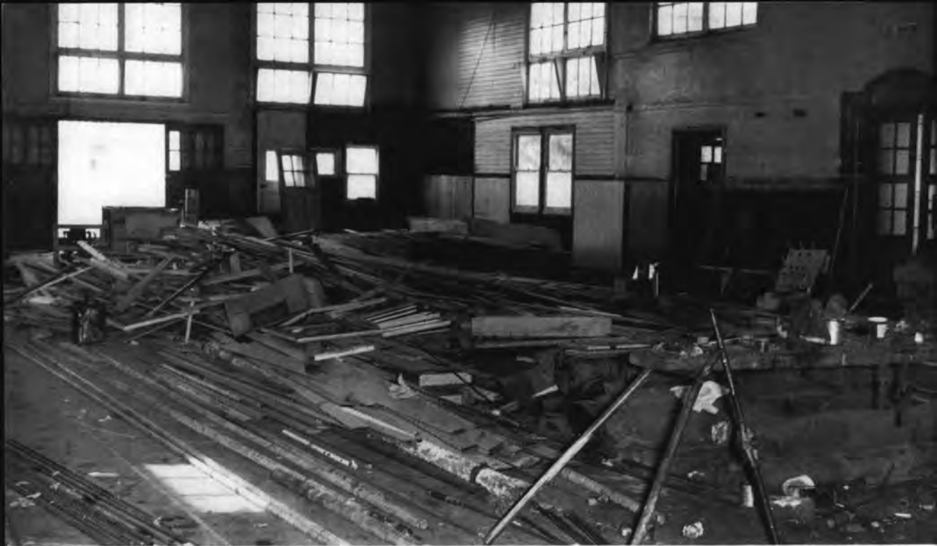
The gymnasium in the process of a face-lift
