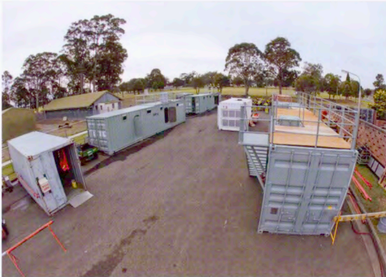
RANSSSS temporary training facility - HMAS Albatross
