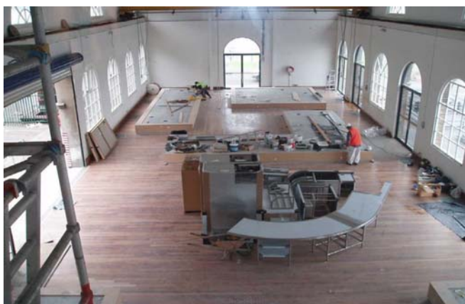
Display plinths under construction in the Gun Mounting Workshop building
