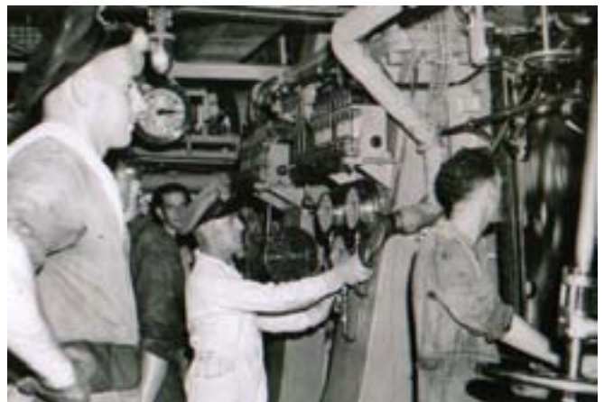
RAN engineers on watch. Temperatures in the engine spaces of a steam-driven warship could typically reach more than 50 °C
