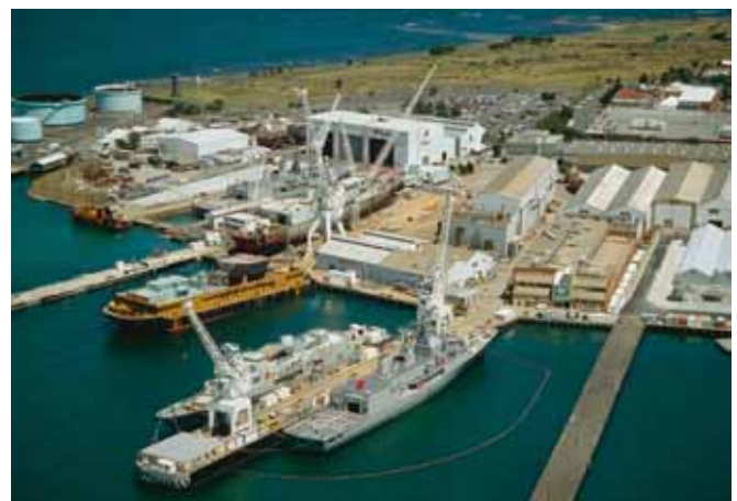
Five Anzac class frigates under construction at the Tenix shipyard at Williamstown, Victoria (Tenix)
