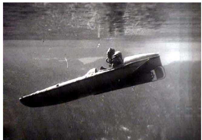
A Sleeping Beauty: a motorised submersible canoe similar to those intended to be used on the RIMAU raid
